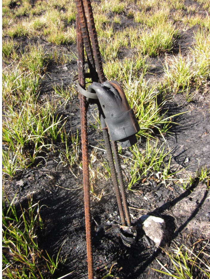
Figure 2-4. Fire-damaged stage recorder in the seasonal pond (dry) on the north side of Poopenaut Valley. This stage recorder was replaced in November 2013.
